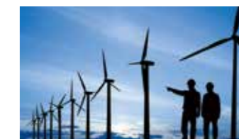
Power Generation Site of Huadian International Ningxia New Energy Power Generation Co., Ltd.
