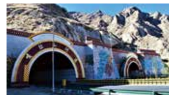
Transportation construction projects in Tibet
